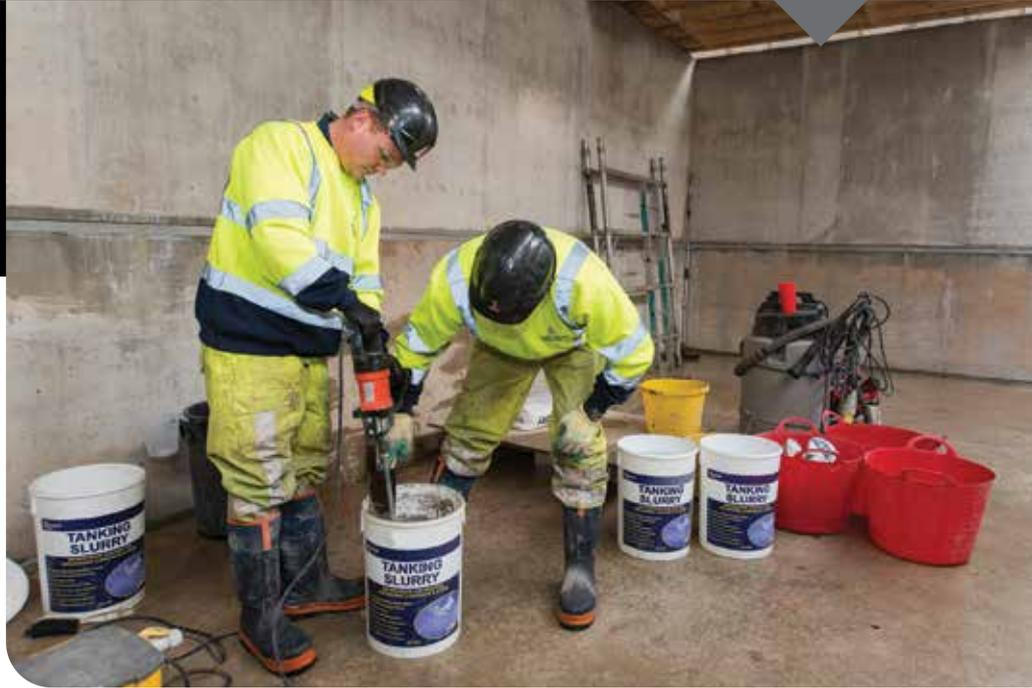
When mixed with clean water and applied correctly, **HydraDry Tanking Slurry** forms a permanent waterproof coating to the concrete and masonry and is easily applied by brush, roller or spray.
