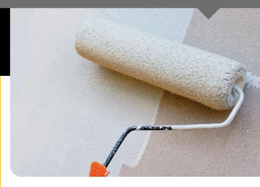
Thermaldry Anti-Condensation Coating is both thermally insulating and water repelling. It increases the wall temperature, thus reducing the 'dew point', or the temperature at which condensation occurs.
